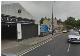
Single Storey Warehouse (to the west side)
